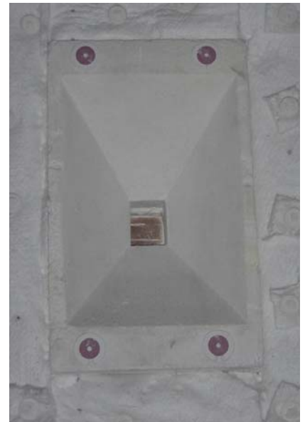
Vacuum formed peephole Installed at BASF - Antwerpen
